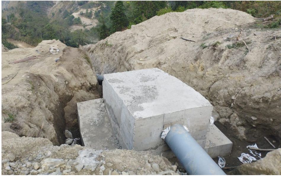
Photo 9-47 Penstock Pipe Anchor Block VAB10
