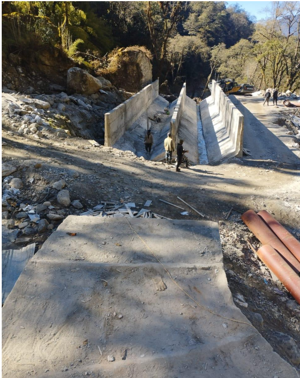
Photo 9-12 Connecting Canal and Desander main chamber
