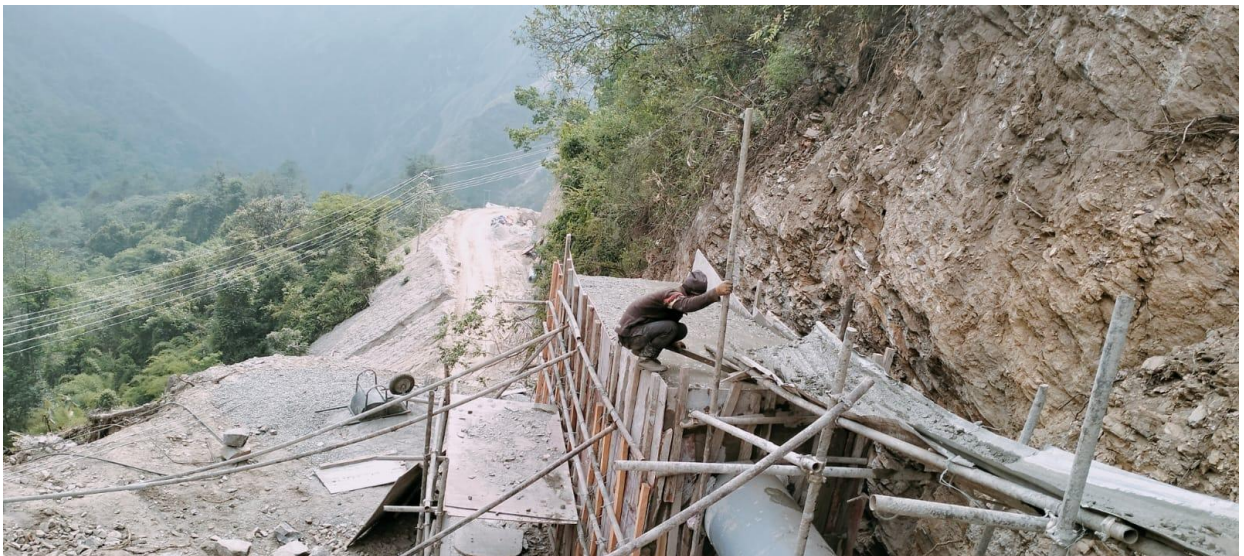
Photo 9-44 Penstock Pipe Anchor Block CAB 22
