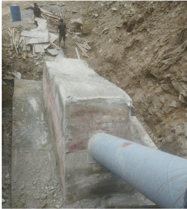
Photo 9-45 Penstock Pipe Anchor Block VAB 07
