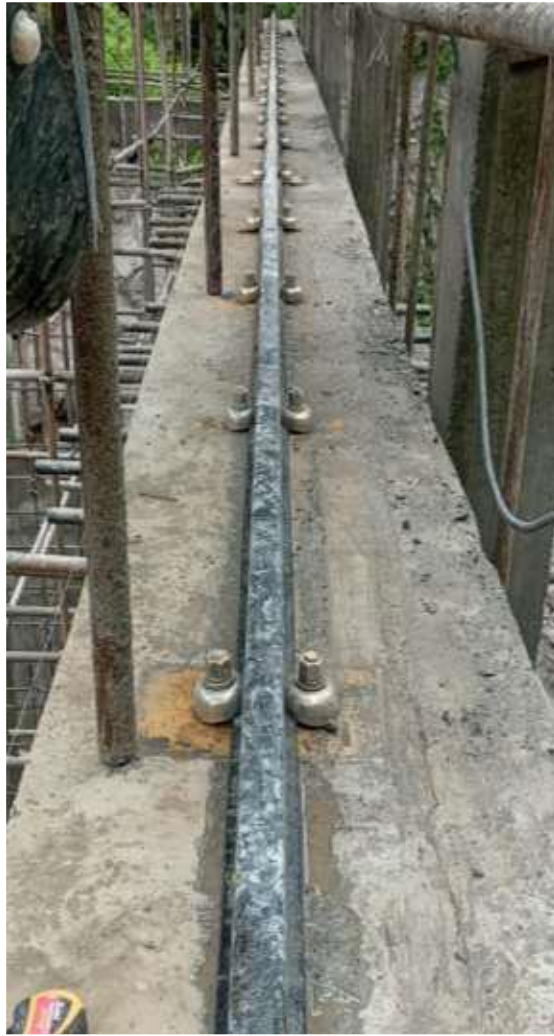
Photo 9-55: Installation of LT rail by EM contractor
