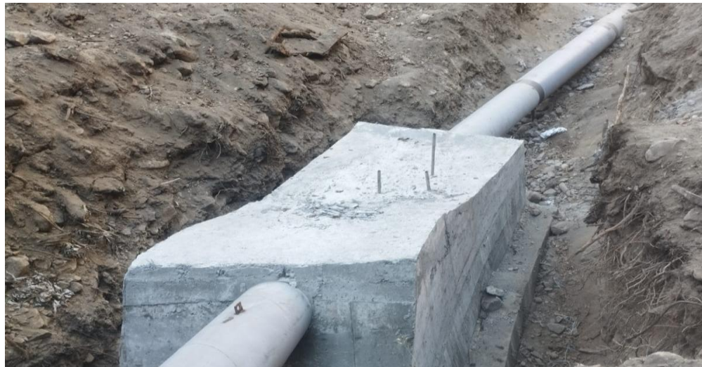
Photo 9-33 Penstock Anchor Block CAB 13
