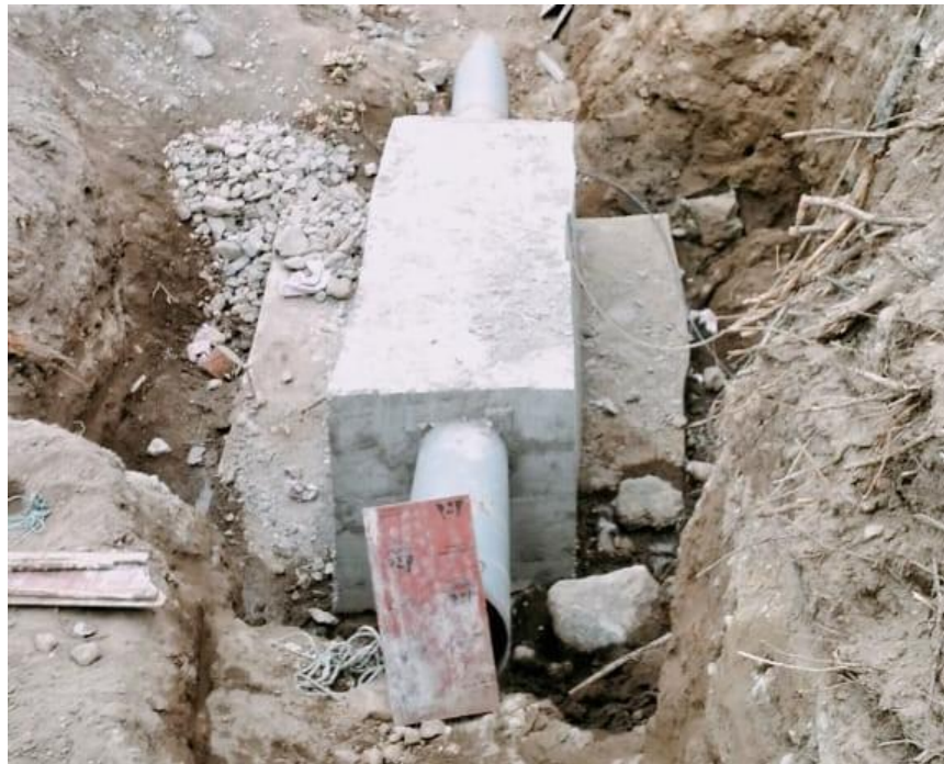
Photo 9-46 Penstock Pipe Anchor Block VAB 09
