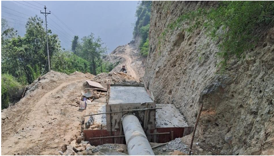
Photo 9-41 Penstock Pipe Anchor Block CAB20
