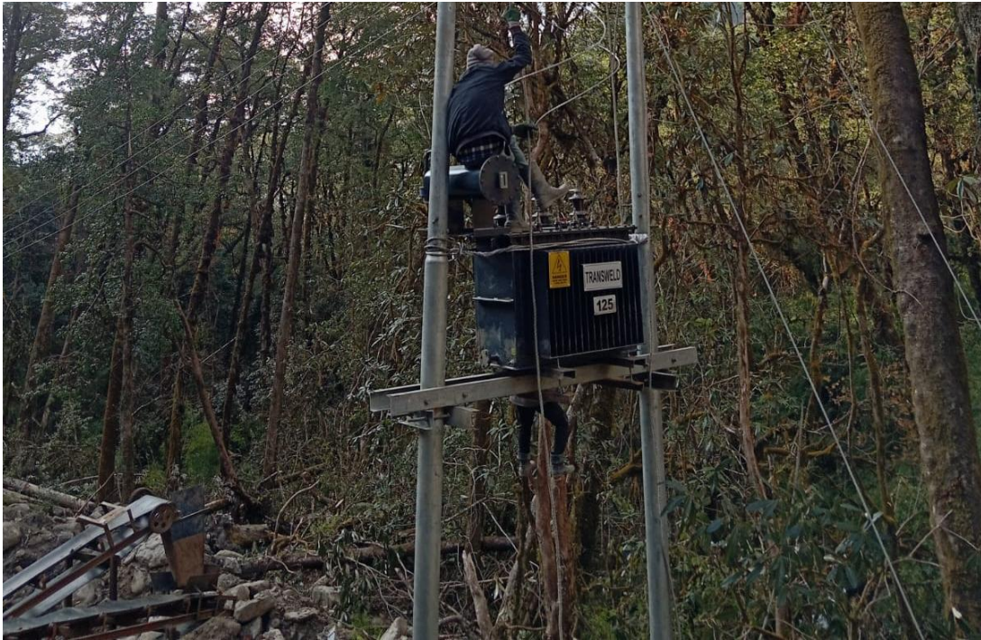
Photo 9-9 Transformer Installation at Intake
