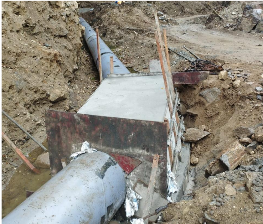
Photo 9-18 Headrace Anchor Block HAB 05
