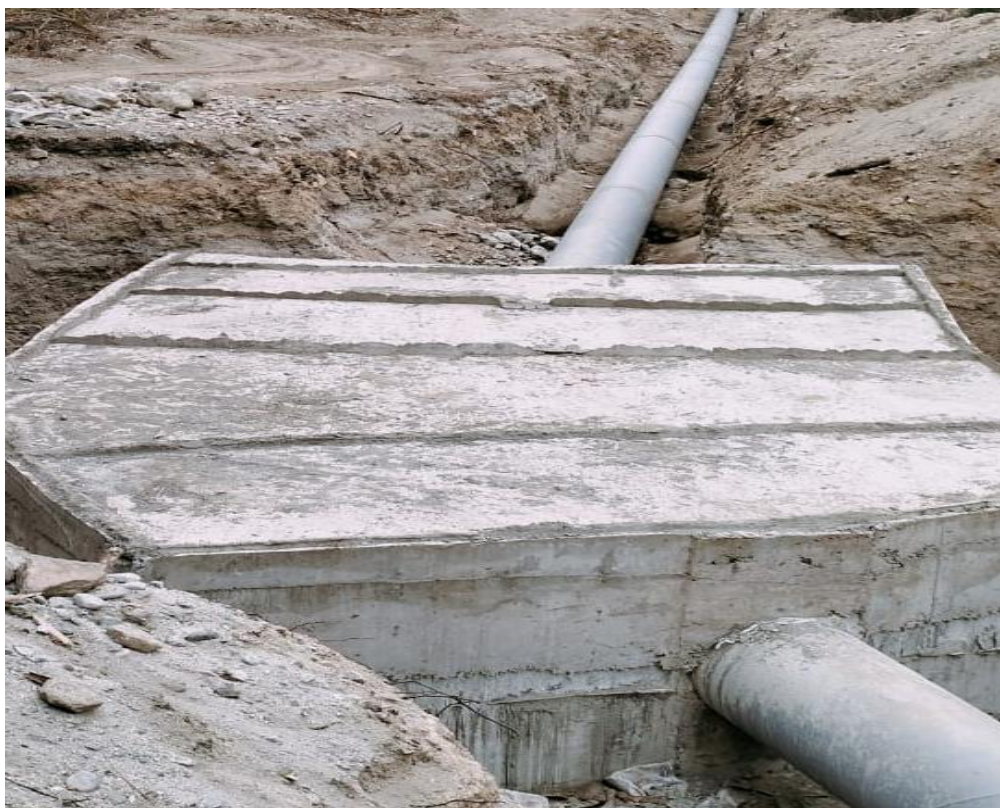
Photo 9-34 Penstock Pipe Anchor Block CAB 14
