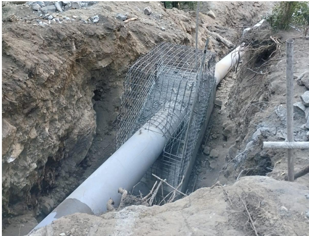
Photo 9-32 Penstock Anchor block VAB2
