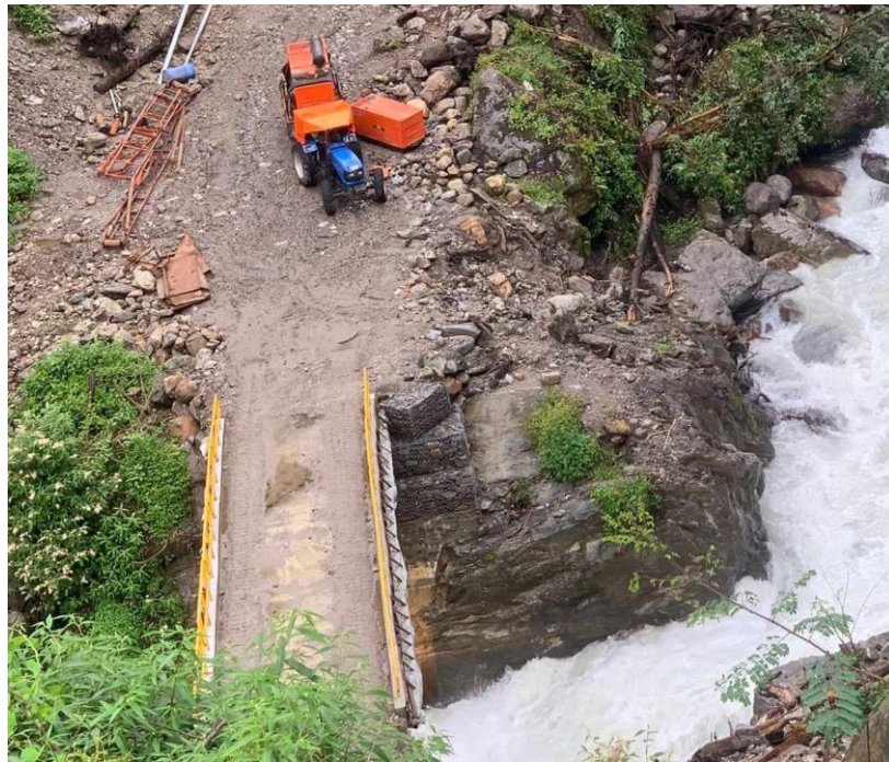
Photo 9-3 Composite steel girder with RCC deck bridge
