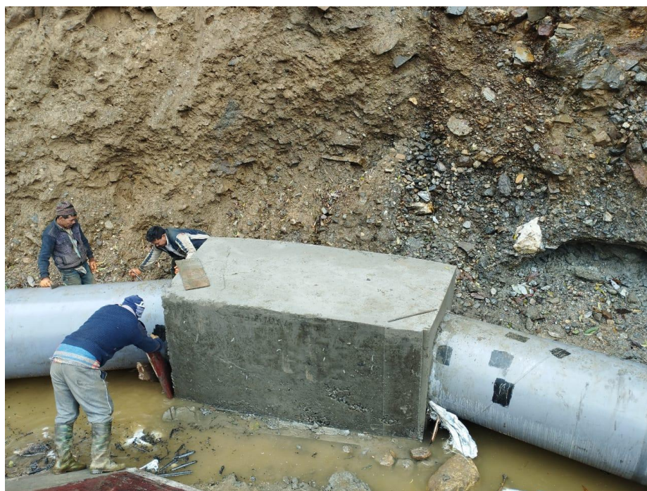
Photo 9-17 Headrace Anchor Block HAB 04
