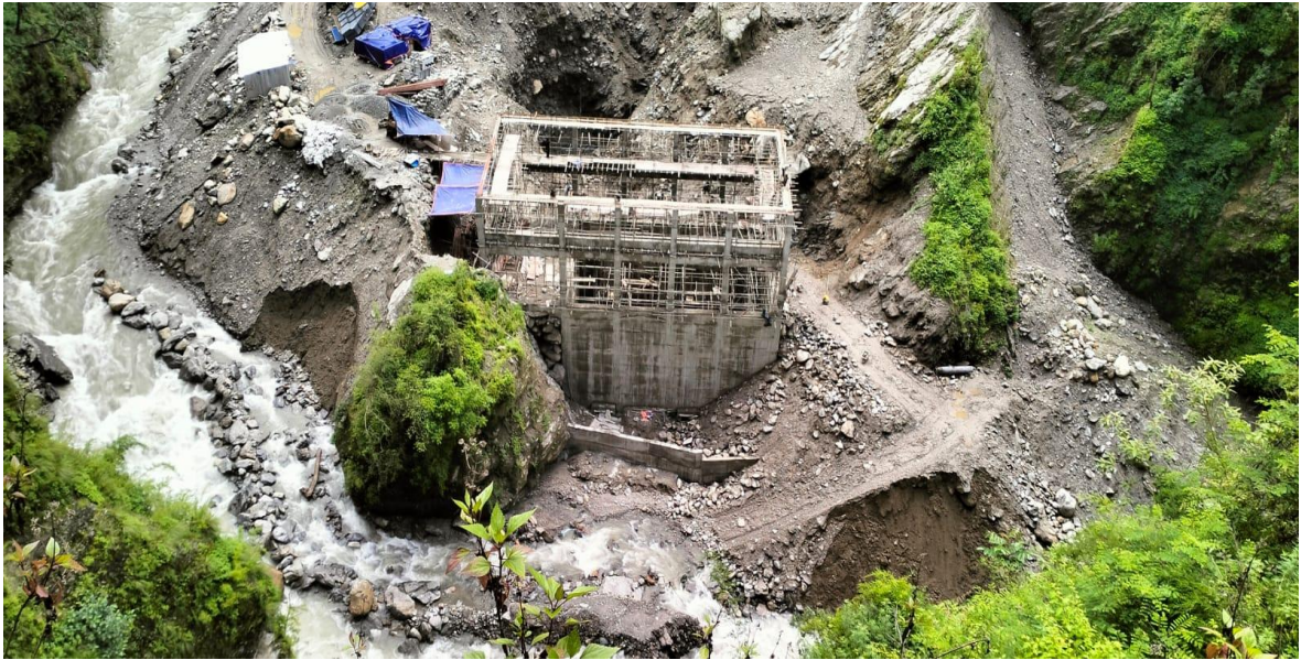
Photo 9-50 Powerhouse superstructure WIP
