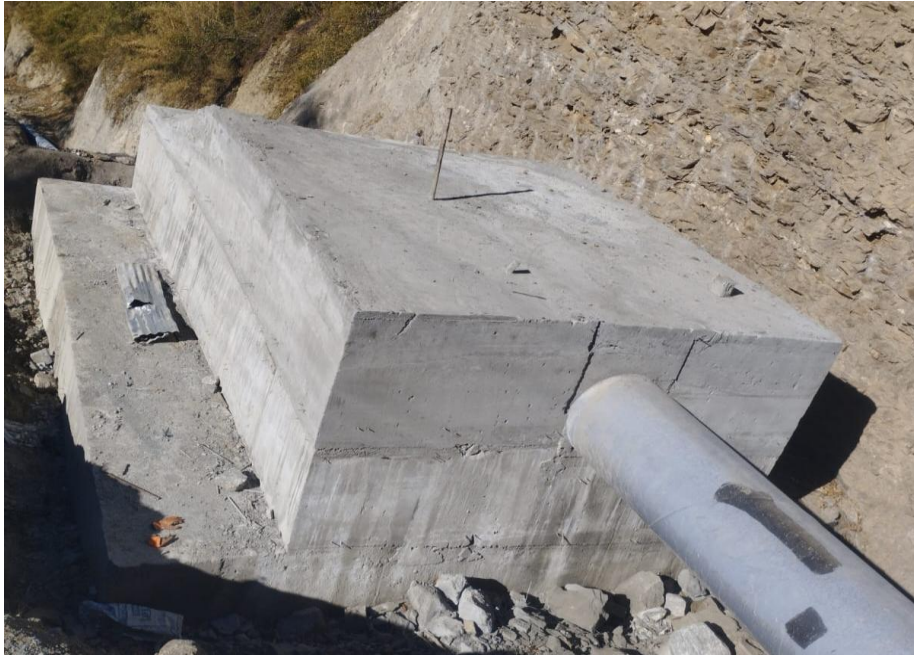
Photo 9-39 Penstock Anchor Block CAB 18
