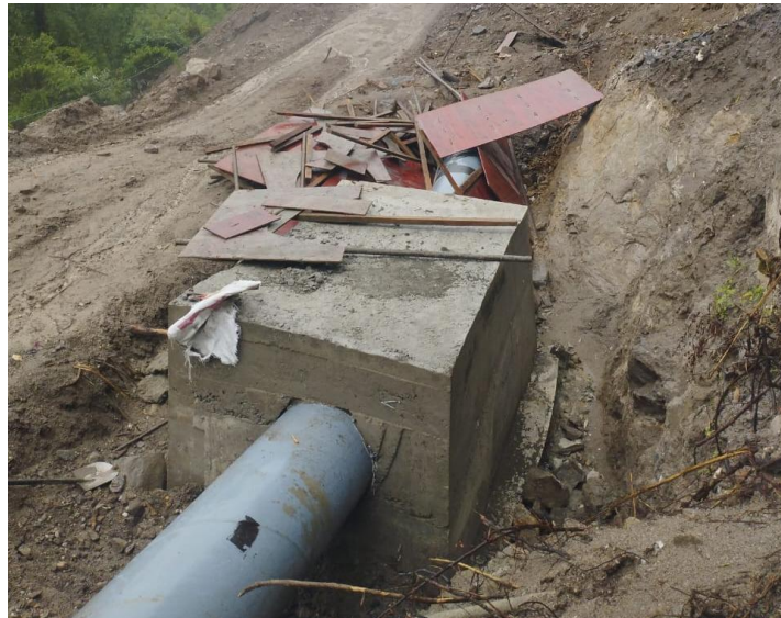
Photo 9-42 Penstock Pipe Anchor Block CAB 21
