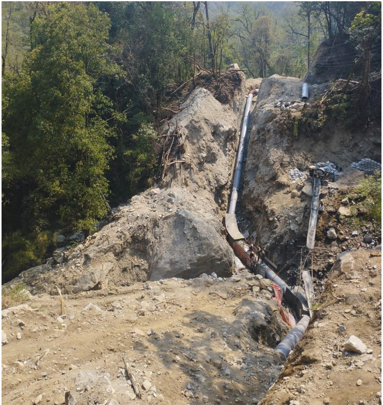
Photo 9-15 Headrace Anchor Block CAB3, CAB4, CAB5 and CAB6 including Siphon crossing
