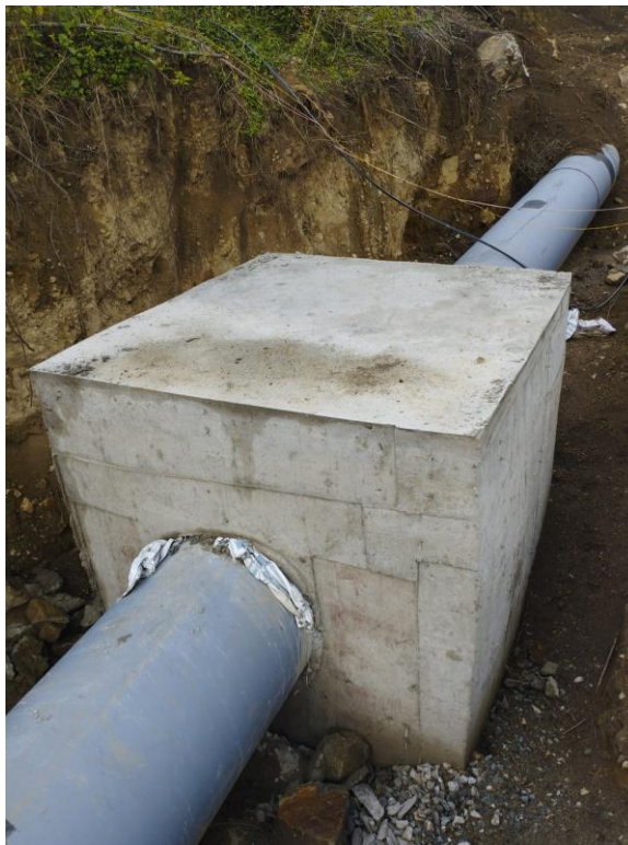
Photo 9-36 Penstock Pipe Anchor Block VAB 04
