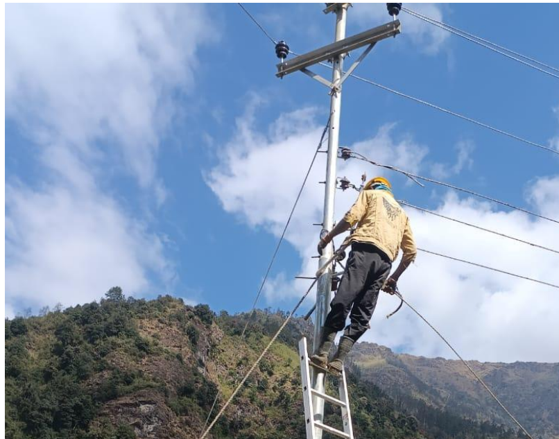
Photo 9-8 Electric Pole and accessories erection for construction power
