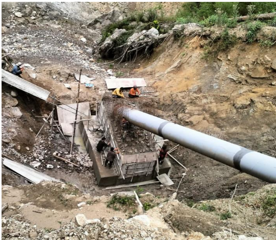
Photo 9-38: Penstock anchor Block CAB 15
