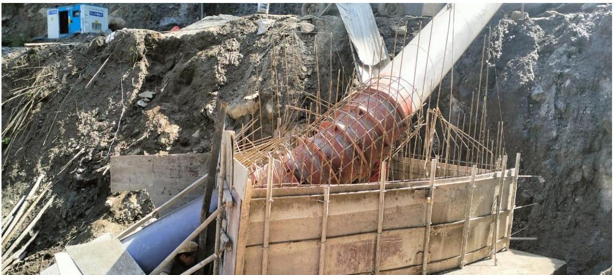
Photo 9-29: Penstock Anchor Block CAB 10
