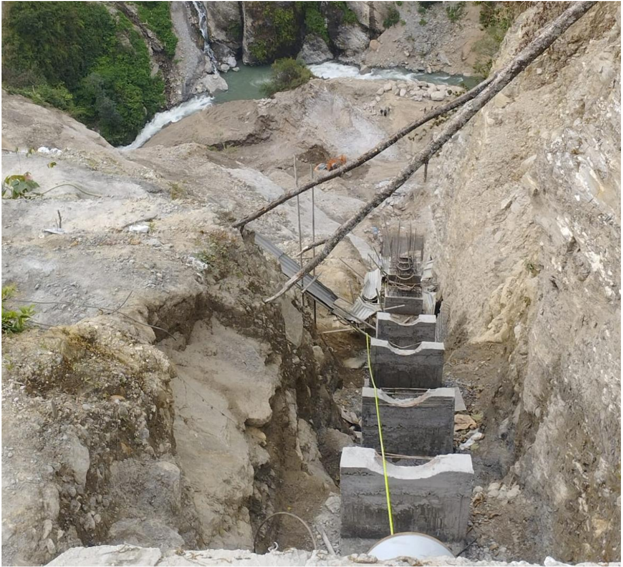
Photo 9-49 Saddle support works from CAB 23 to VAB11
