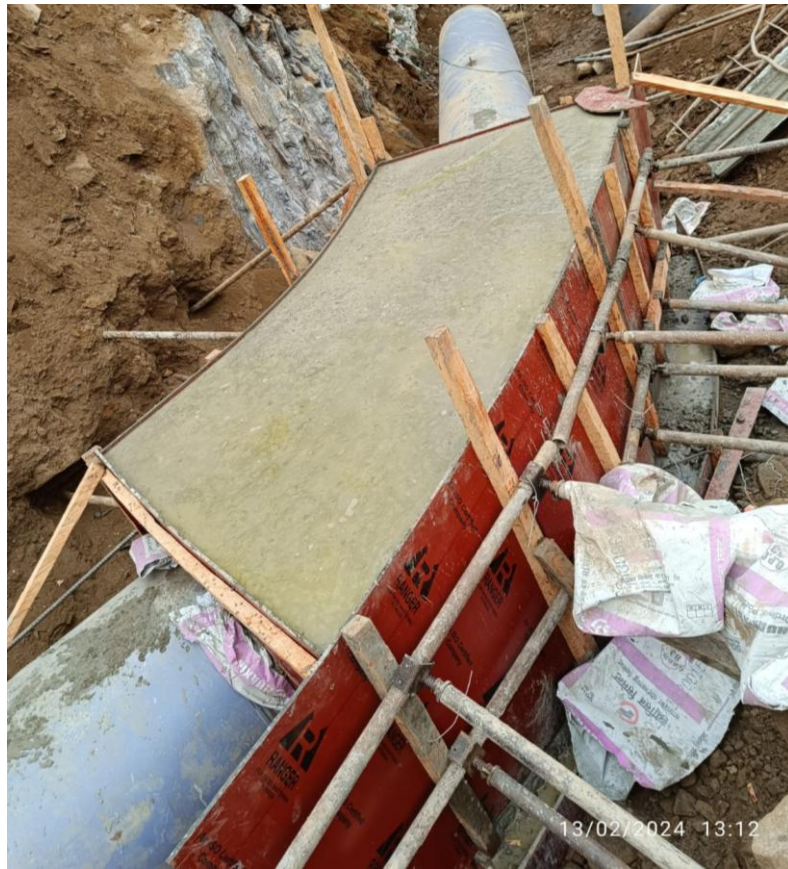
Photo 9-20 Headrace Anchor Block HAB07
