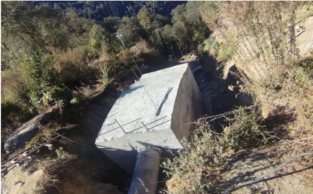
Photo 9-37 Penstock Anchor Block VAB 5
