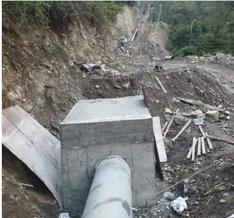
Photo 9-43 Penstock Pipe Anchor Block VAB 06
