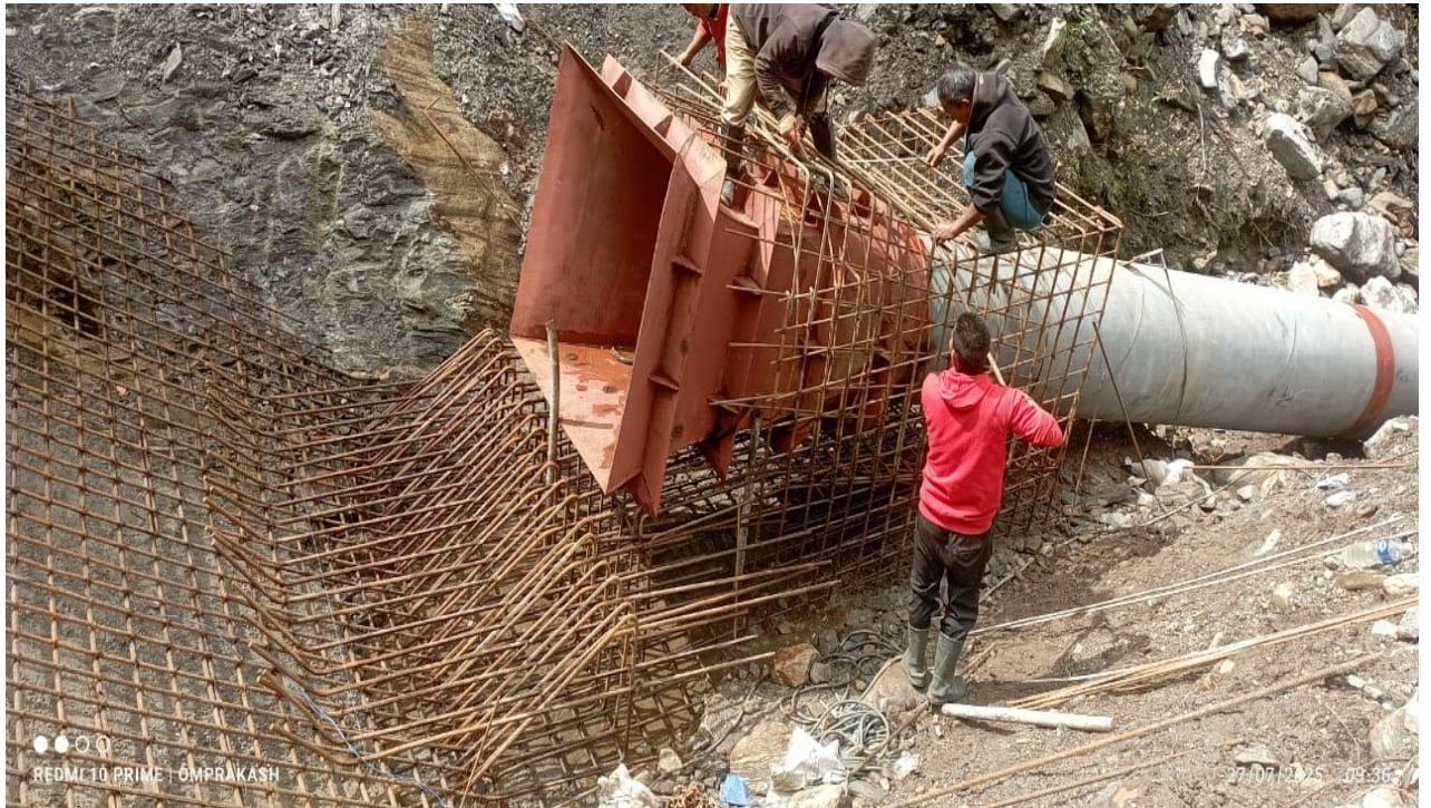
Photo 9-48 Rebar work of bellmouth completed.
