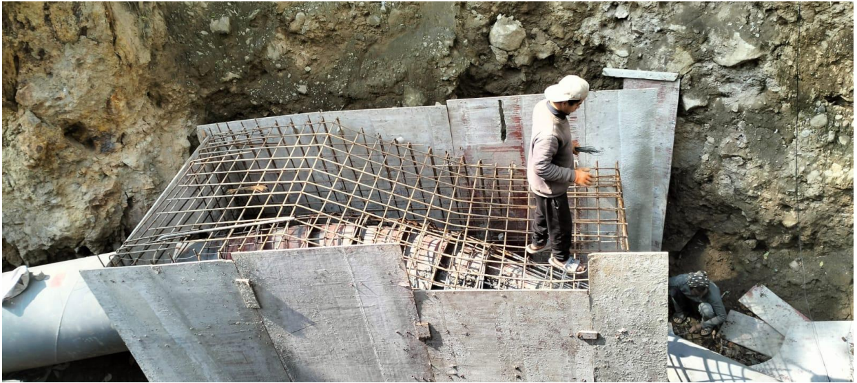
Photo 9-28 : Penstock Anchor Block CAB8
