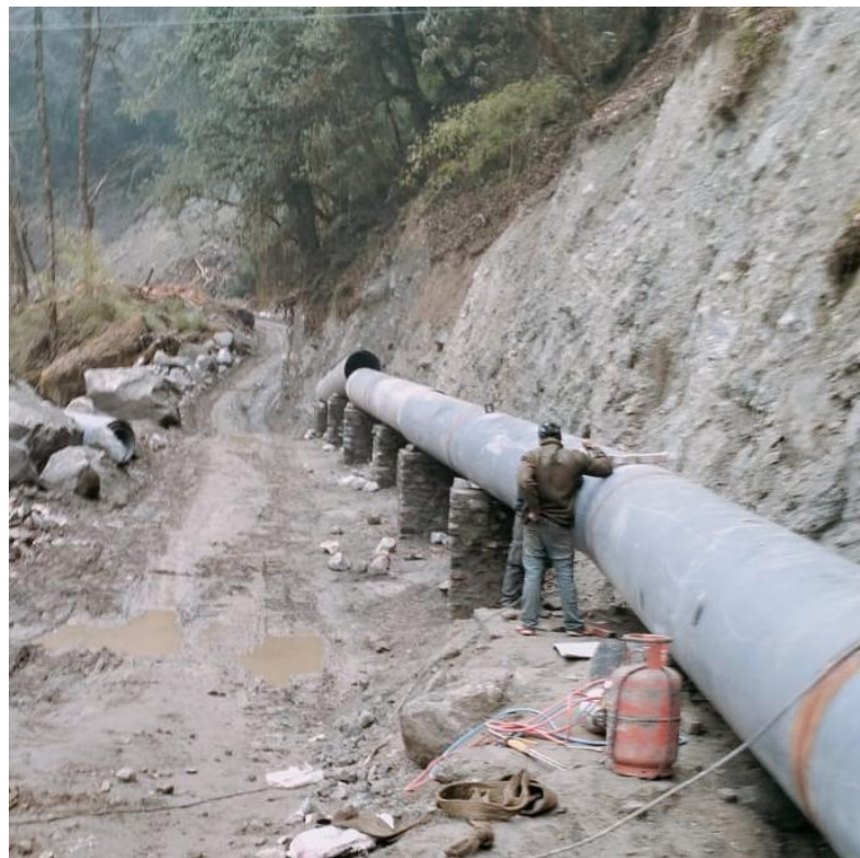
Photo 9-14 Headrace Pipe erection near HAB 02
