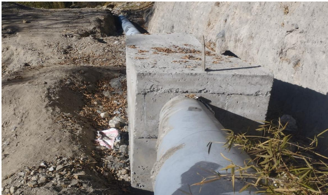
Photo 9-40 Penstock Anchor Block CAB19
