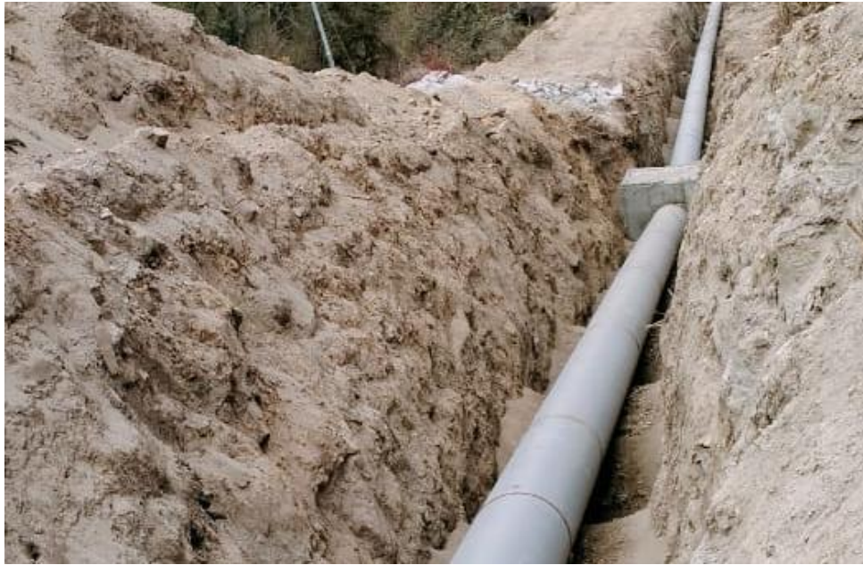
Photo 9-35 Penstock Pipe Anchor Block VAB 03
