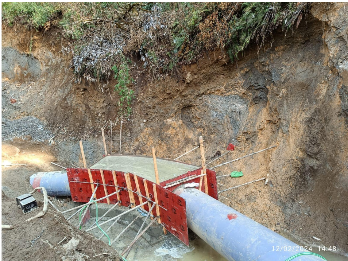
Photo 9-24 Headrace Pipe Anchor Block HAB 11
