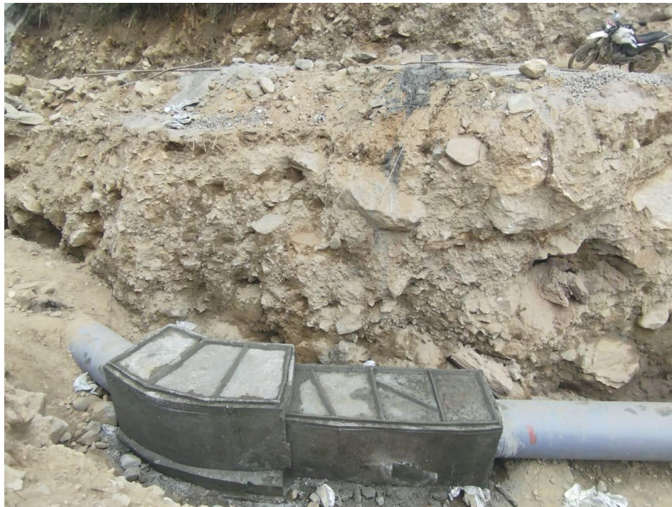
Photo 9-16 Headrace Anchor Block HAB 03 and Road crossing
