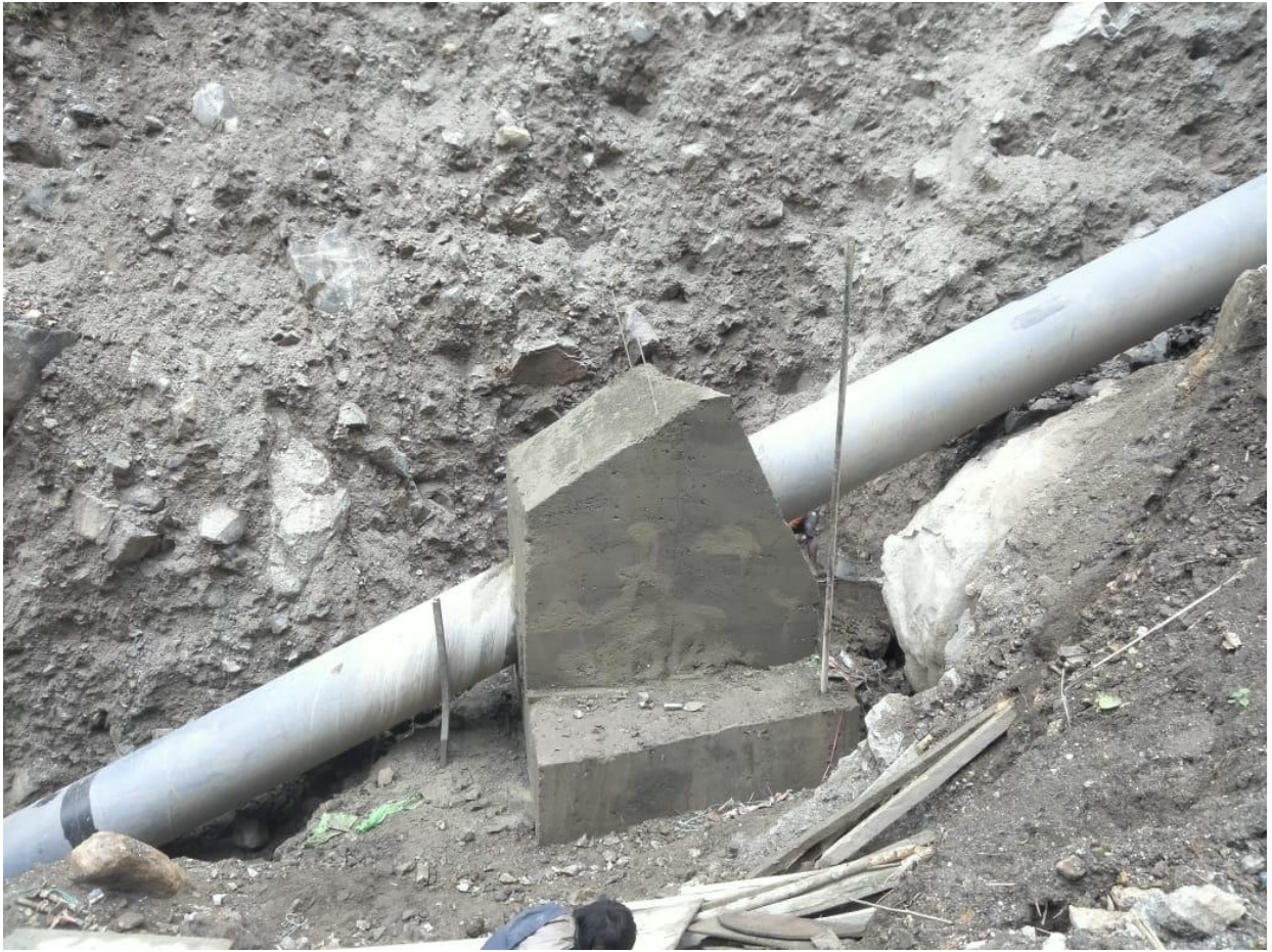
Photo 9-30: Penstock Anchor Block VAB 1
