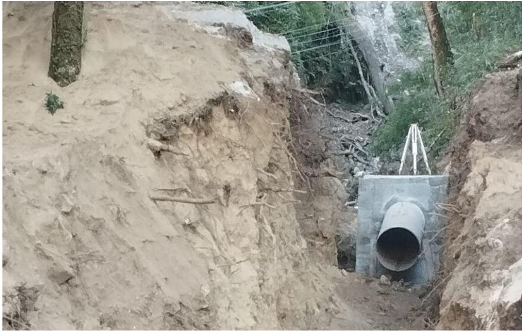
Photo 9-31 Penstock anchor block CAB 12
