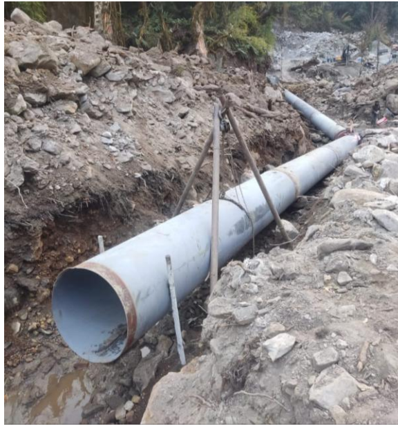
Photo 9-13: Headrace Pipe from Bellmouth to CAB 1 to CAB 2
