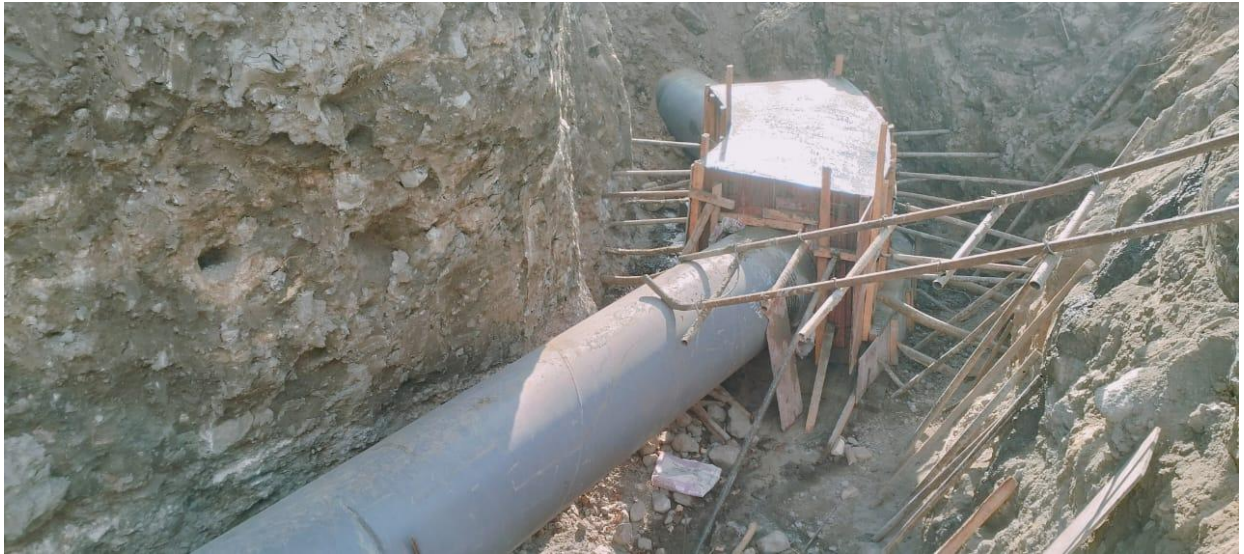
Photo 9-23 Headrace Pipe anchor block HAB 10
